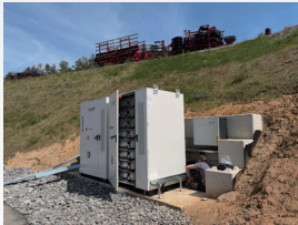
Germany OASIS L344 & Kaco 184kW/688kWh Outdoor-Batterieschrank
