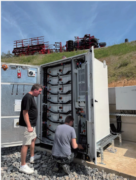
Germany OASIS L344 & Kaco 184kW/688kWh Outdoor-Batterieschrank
